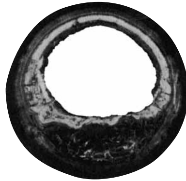
1/2 inch scale in 6 inch pipe, 1000 feet long, has a transfer capacity loss of 150 gallons per minute.
